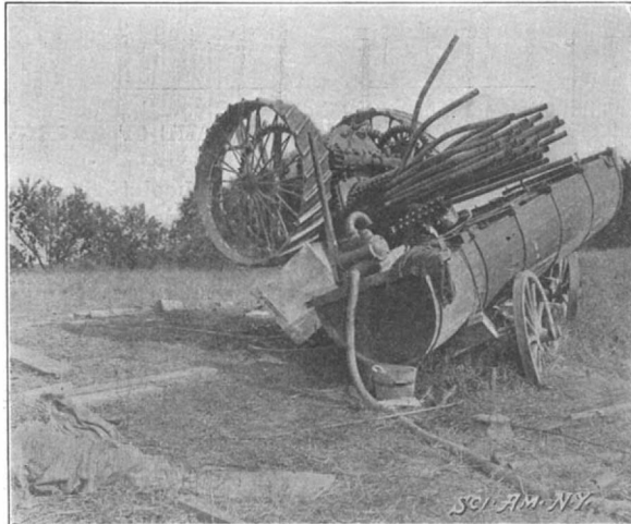
FIREBOX AND TUBES THROWN OVER AND BACK UPON TENDER.
