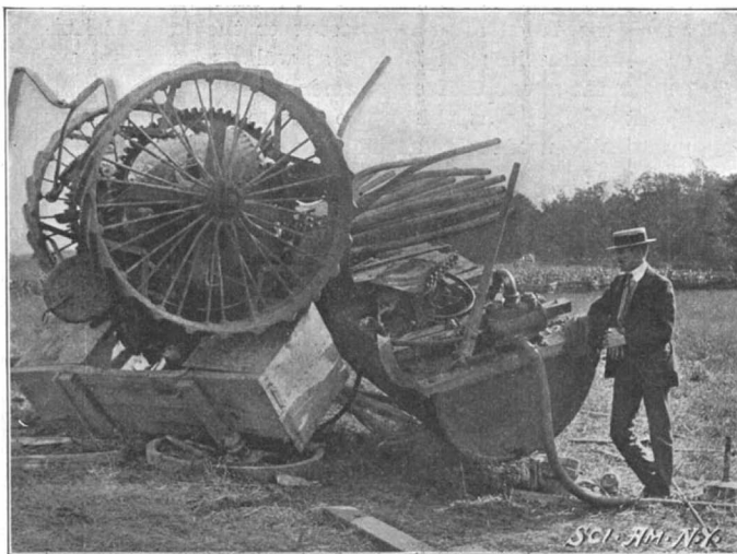
PORTABLE ENGINE BOILER EXPLOSION.
