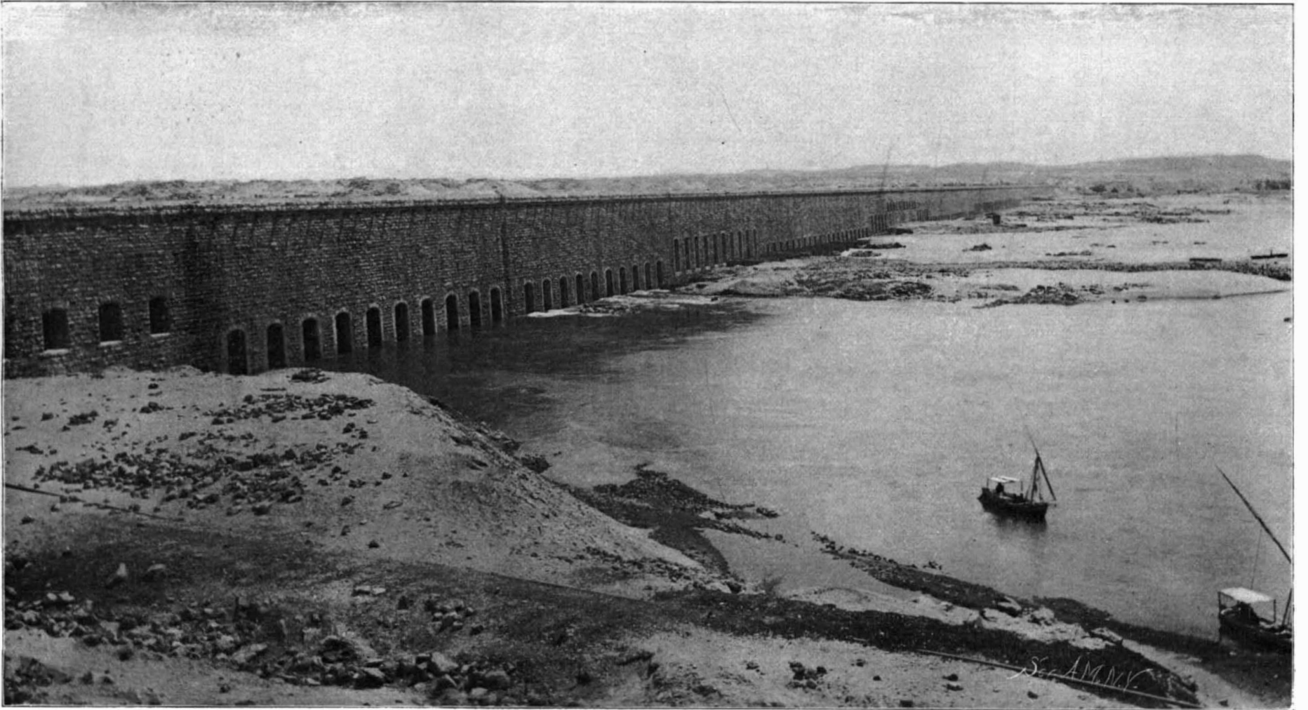
Total length, 1\frac{1}{4} miles; maximum height above foundation, 130 feet; difference of water level above and below, 67 feet. Total weight of masonry, over 1,000,000 tons. South, or Upstream Side of Dam from West Bank.
