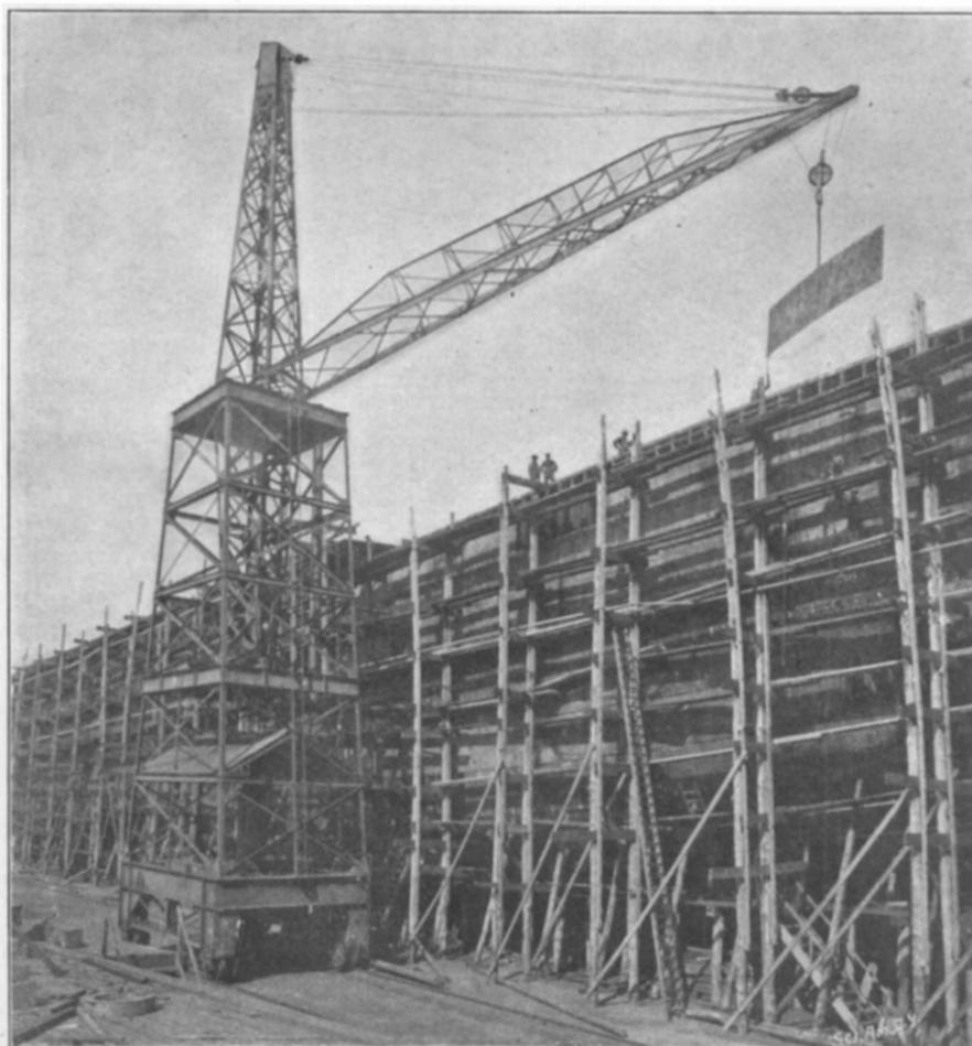
Locomotive Derrick Crane with Single Boom of Latticed Steel Construction.
