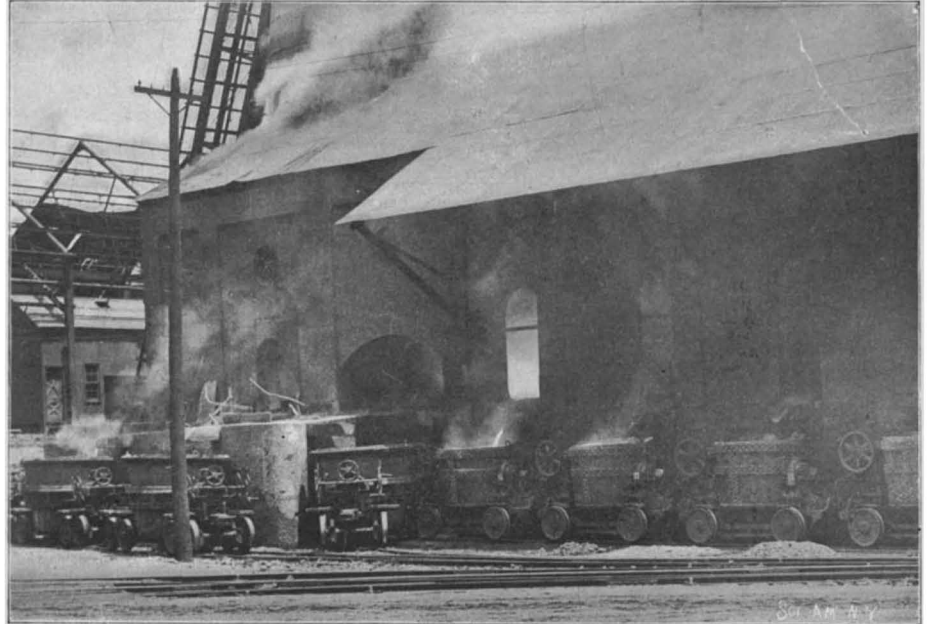
Tapping Contents of Blast Furnace Into Ladles.
