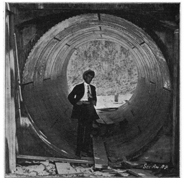
INSIDE PENSTOCK—9 FEET IN DIAMETER.
