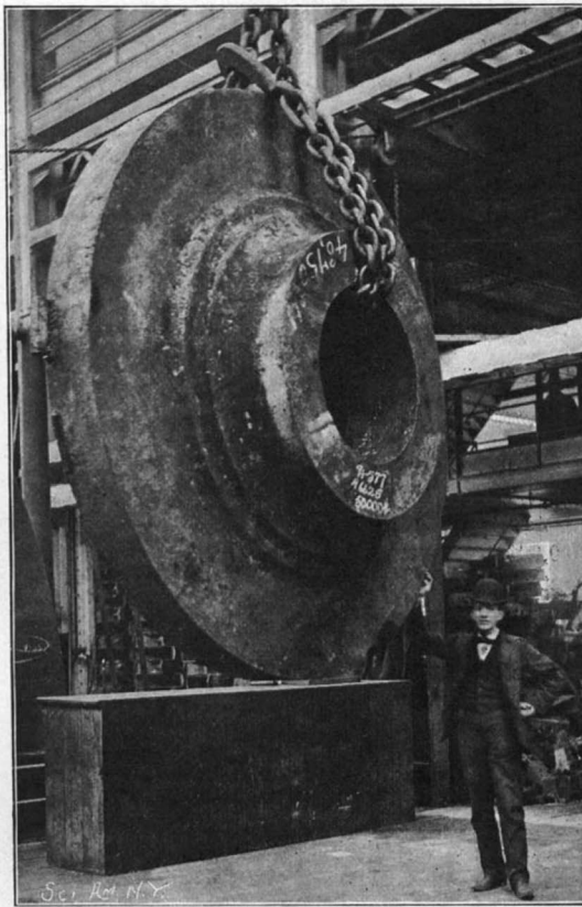
Massive Steel Hub Casting for the Field of the Westinghouse Alternator; Weight 25 Tons.
