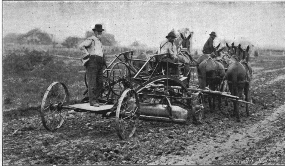
Road Scraper at Work.
