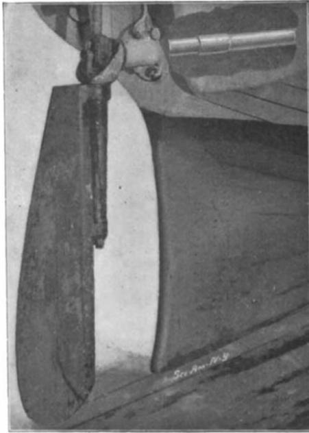
**PENDULUM PROPELLER DRIVING FORWARD, SHOWING SHAFT.**
