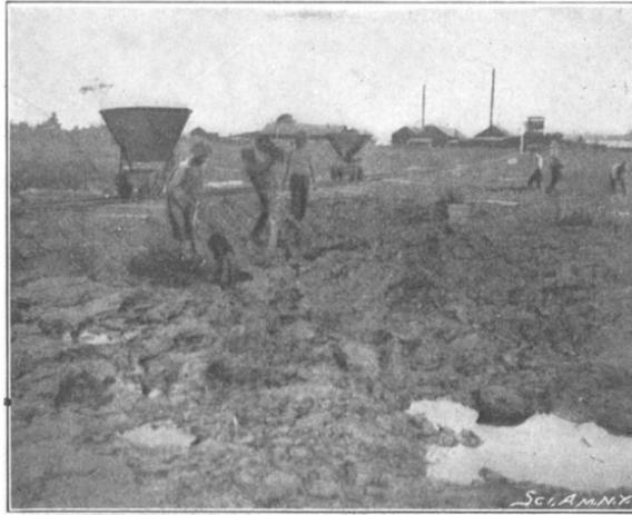
DIGGING AND LOADING ASPHALT ON THE LAKE.
