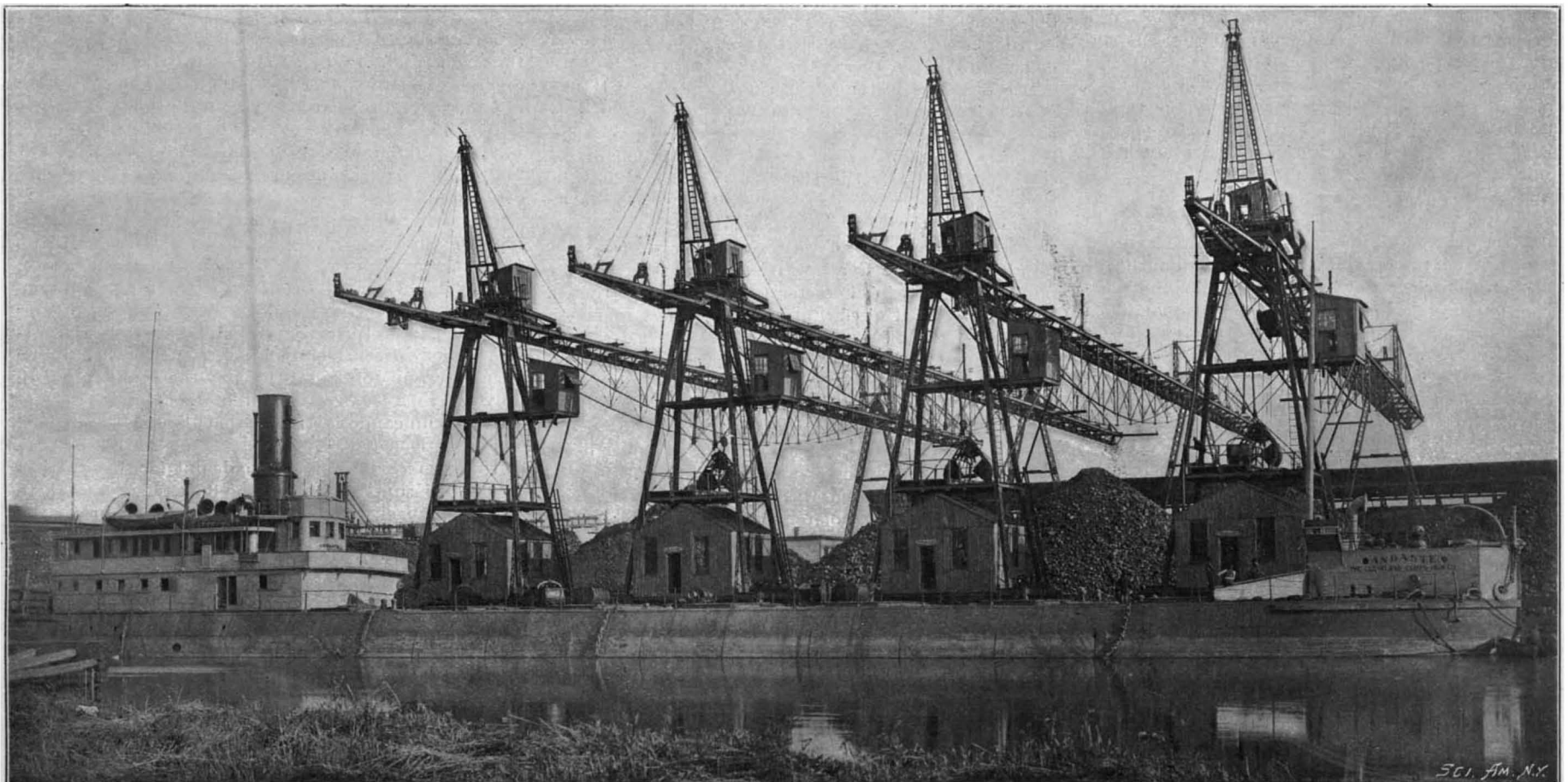
Four-Bridge, Coal Frameway for Unloading Anthracite.
