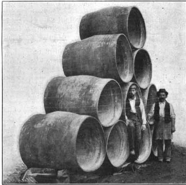
File of Huge Dredging Sleeves, Used as Flexible Connections Between the Pontoons that Carry Dredging Pipes.
