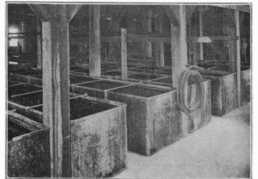
Tanks Dissolving the Borate of Lime
