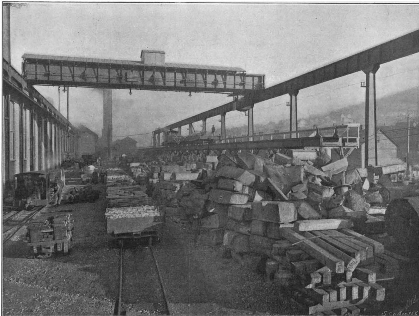
The scrap from the various forges and machine shops is brought to this yard, and stacked according to its chemical composition. Here the "mixture" is made up in boxes and carried on cars to the open hearth furnaces.
