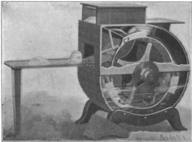
Fig. 1.—AN AUTOMATIC DISH-WASHER.
