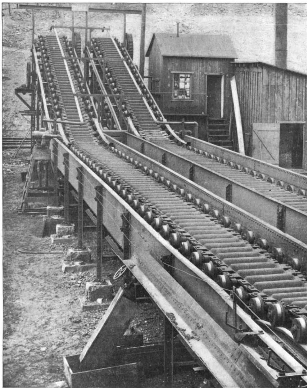
View of Casting Machine, Showing Moulds and Tank Empty and Submerging Device.
