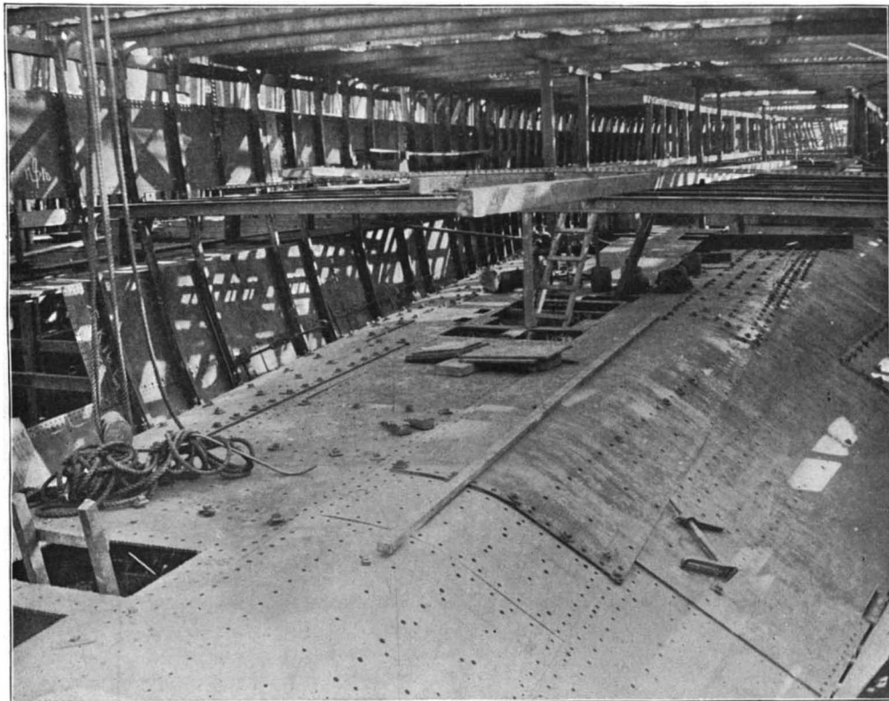
5.—Armored Deck Plated in; Side Framing Carried to Main Deck.
