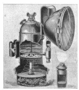
ACETYLENE LAMP, WITH FILTER.
