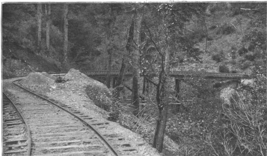
1.—A TYPICAL CURVE AND TRESTLE.
