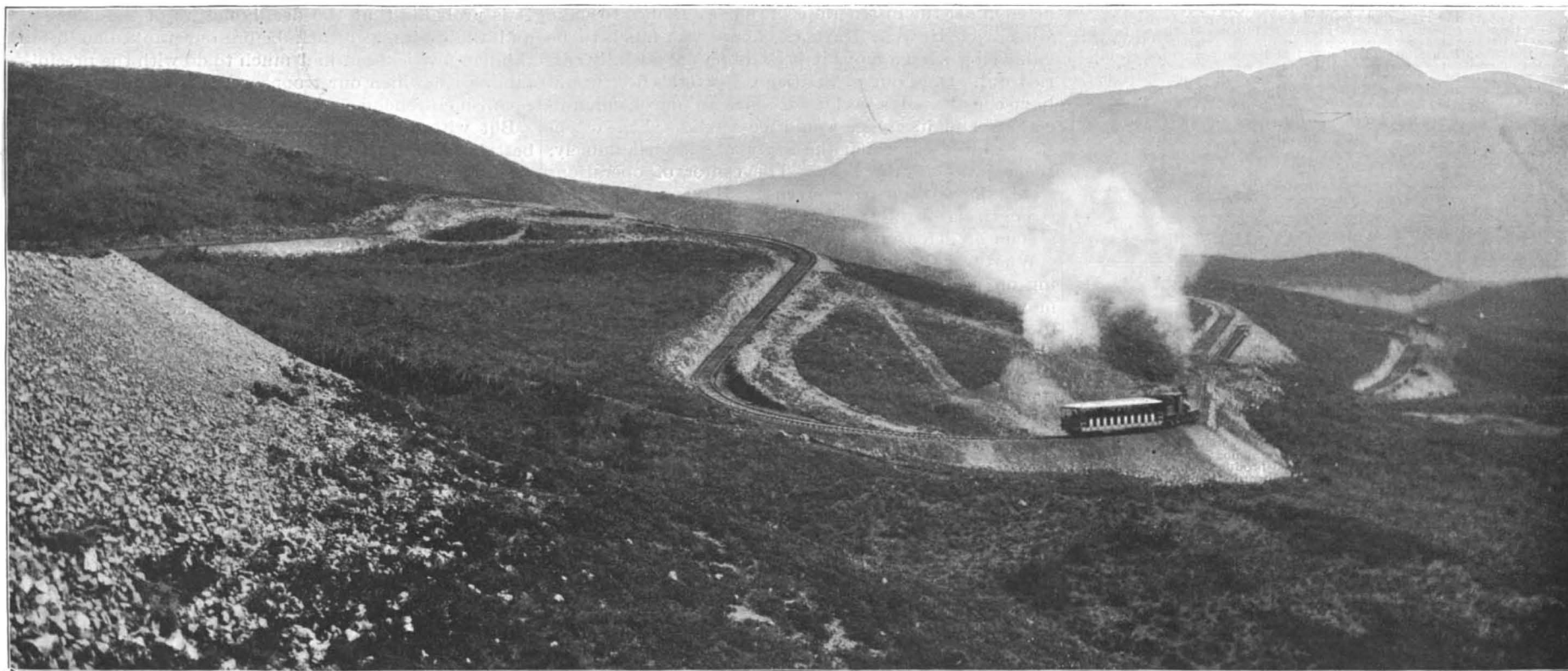
3.—THE "DOUBLE BOW KNOT"—TRACK PARALLELS ITSELF FIVE TIMES.
