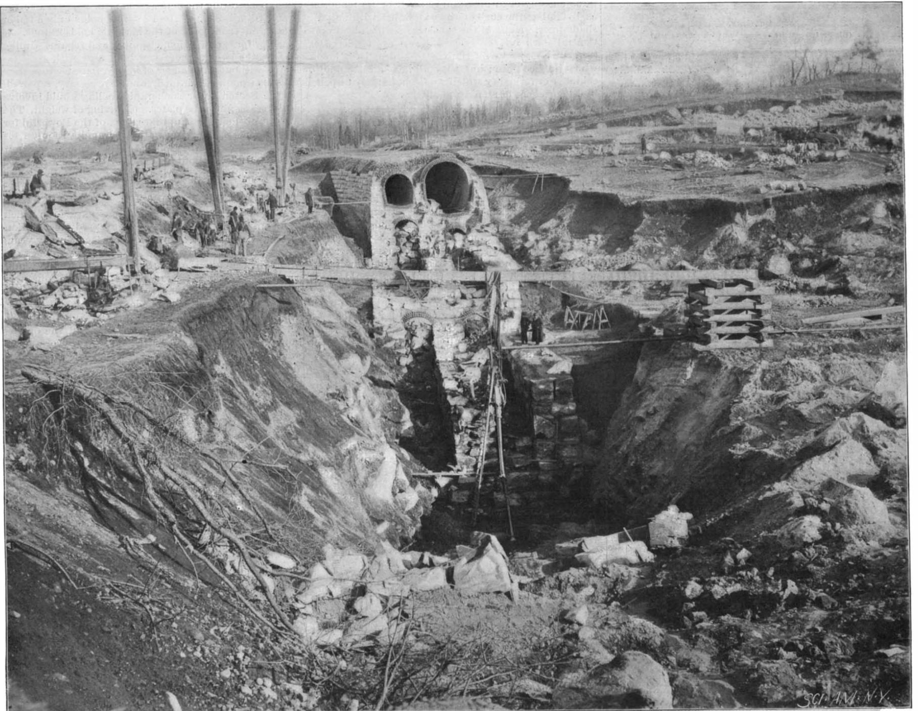
DOUBLE CONDUIT FOR CARRYING WATERS OF OLD AND NEW AQUEDUCTS INTO RESERVOIR. BOTTOM OF EXCAVATIONS IS AT LEVEL OF FINISHED FLOOR OF RESERVOIR. THE WATER SUPPLY OF NEW YORK CITY—JEROME PARK RESERVOIR.—[See page 314.]
