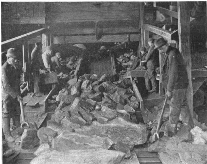
Fig. 1.—CLEARING THE LUMP COAL FROM THE HOISTING SHUTE.
