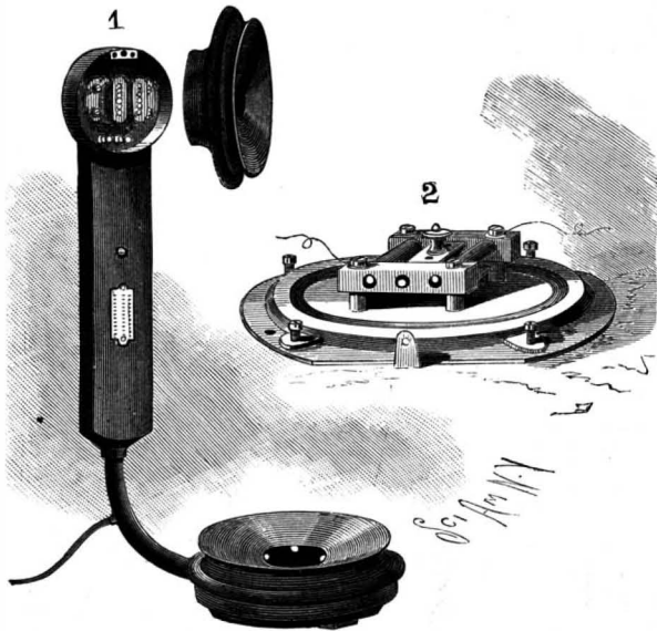
NORIEGA'S COMBINED TELEPHONE RECEIVER AND TRANSMITTER.
