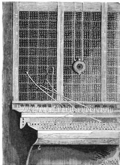
Fig. 2.—ARRANGEMENT OF SPRING JACKS, SWITCHES, AND ANNUNCIATORS ON SWITCHBOARD.
