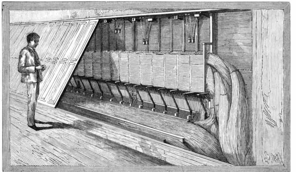
Fig. 3.—REAR VIEW OF SWITCHBOARD, SHOWING CABLES.
