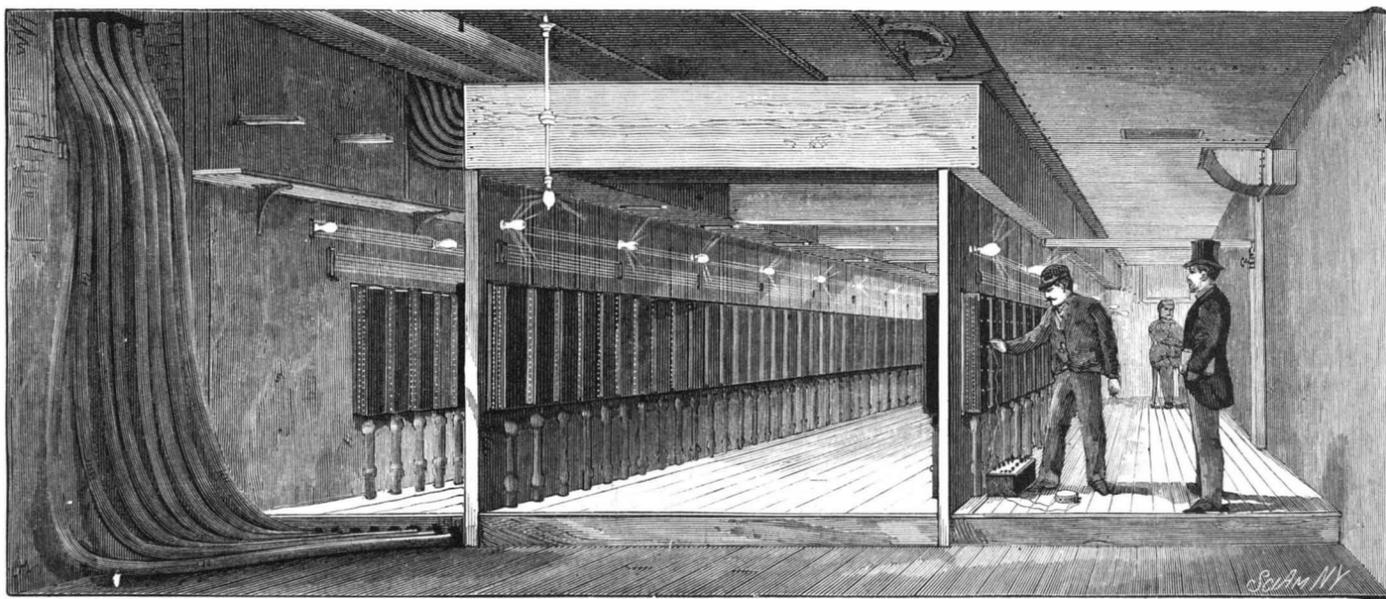
Fig. 7.—TESTING ROOM AND CONNECTION BOXES FOR SWITCHBOARD.
