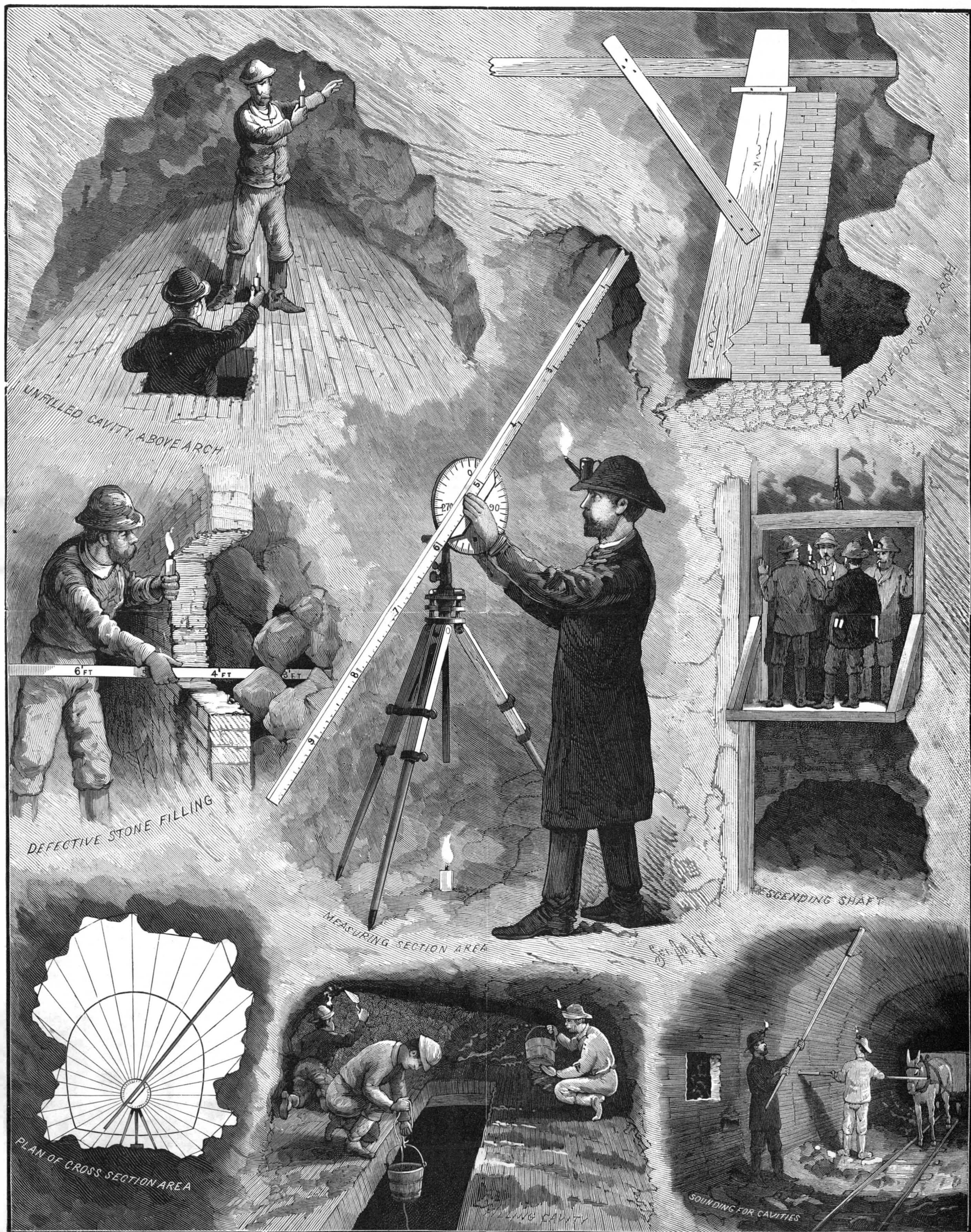
IRREGULARITIES IN THE CONSTRUCTION OF THE NEW YORK AQUEDUCT.—[See page 6.]
