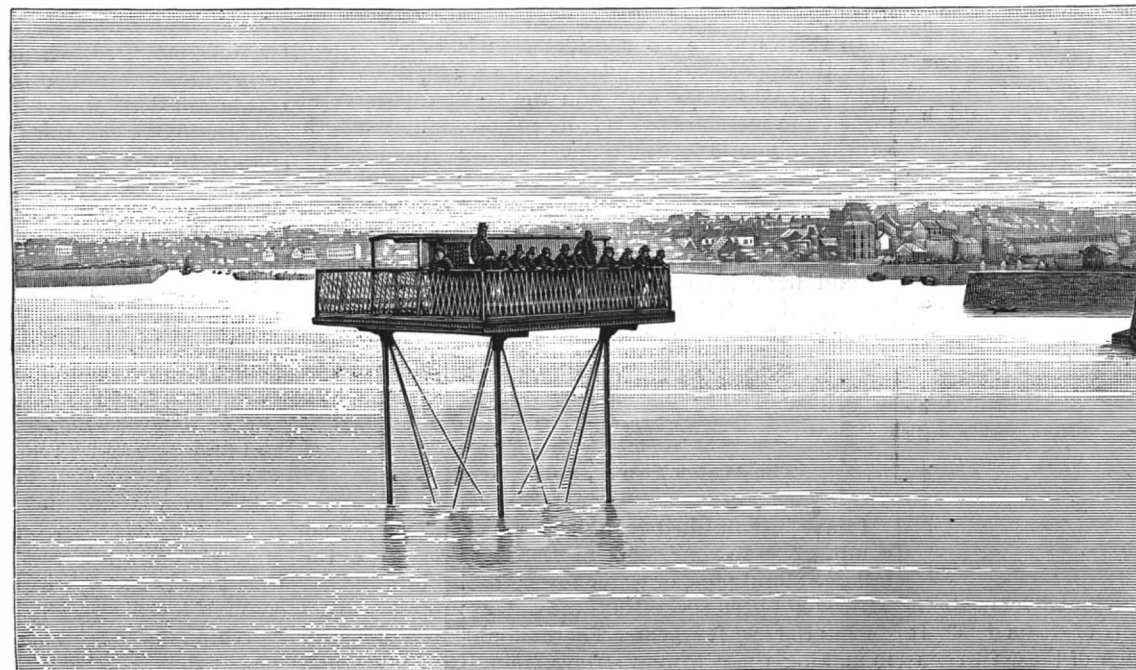
Fig. 2.—THE SAINT MALO ROLLING BRIDGE AT HIGH TIDE.
