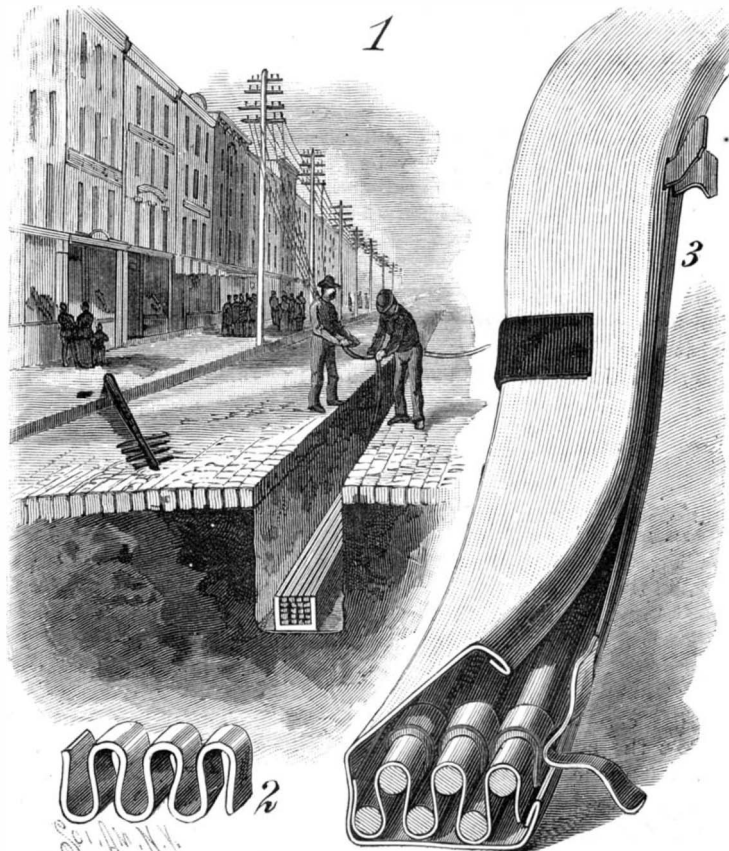
McGILL'S INSULATOR FOR ELECTRICAL CONDUCTORS.
