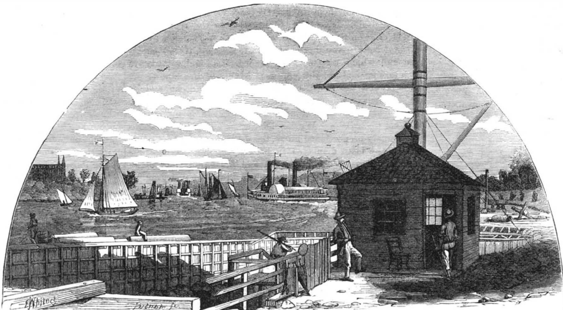
VIEW OF HELL GATE FROM TOP OF COFFER DAM.
