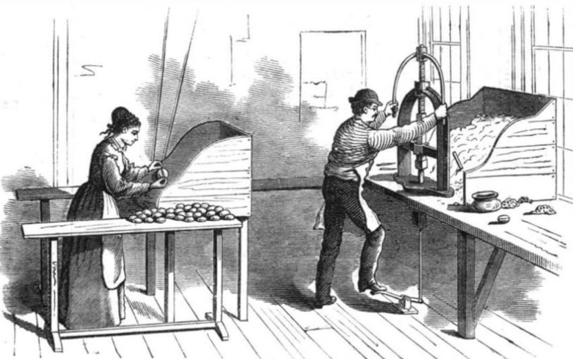
Fig. 2.—PRESSING AND TURNING SMALL WARE.
