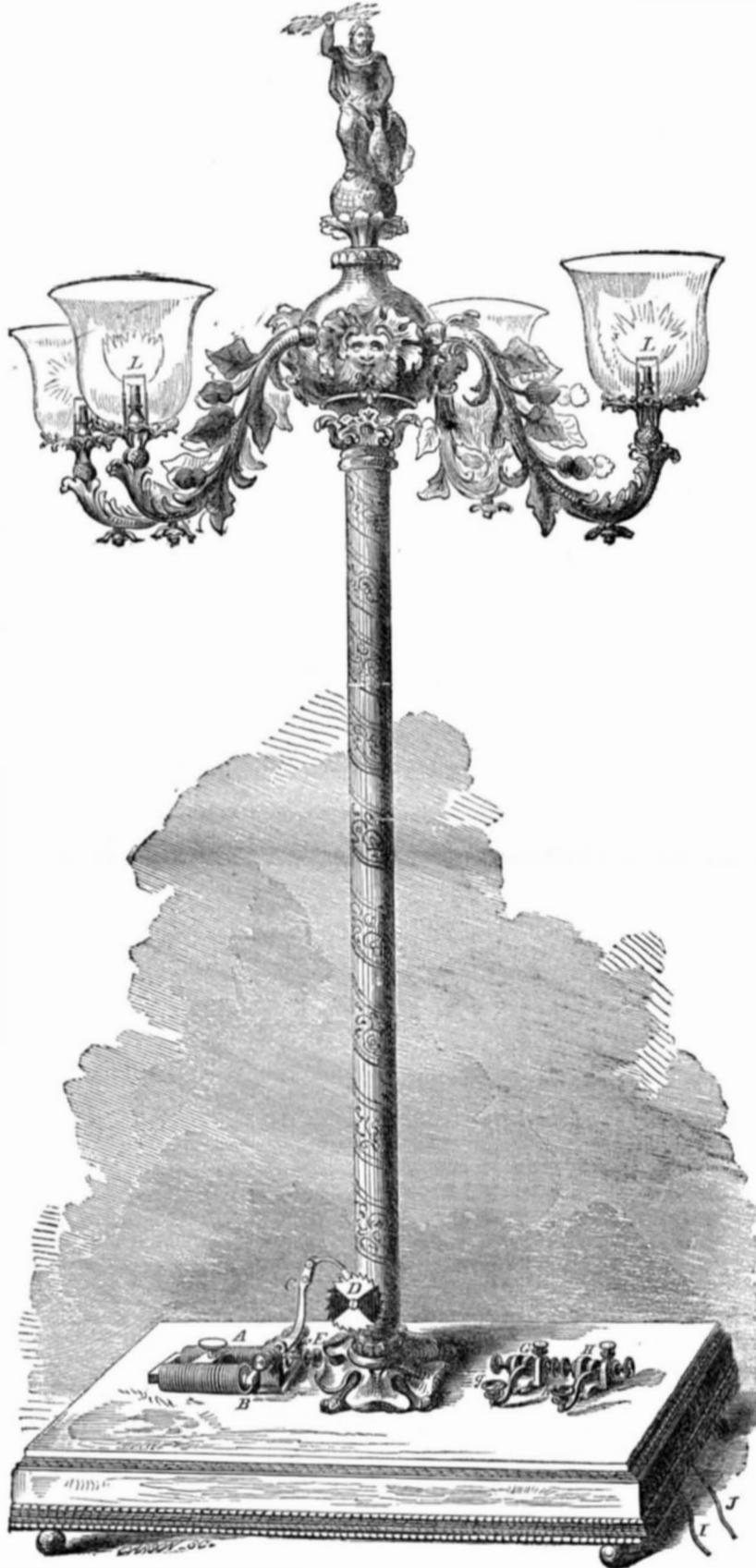
which, as ordinarily conducted, occupies two men an hour. As a means of showing its power, it is customary to shut off and again ignite the gas between each act. The battery employed is Smee's, thirty cups being employed, each of one gallon capacity.
