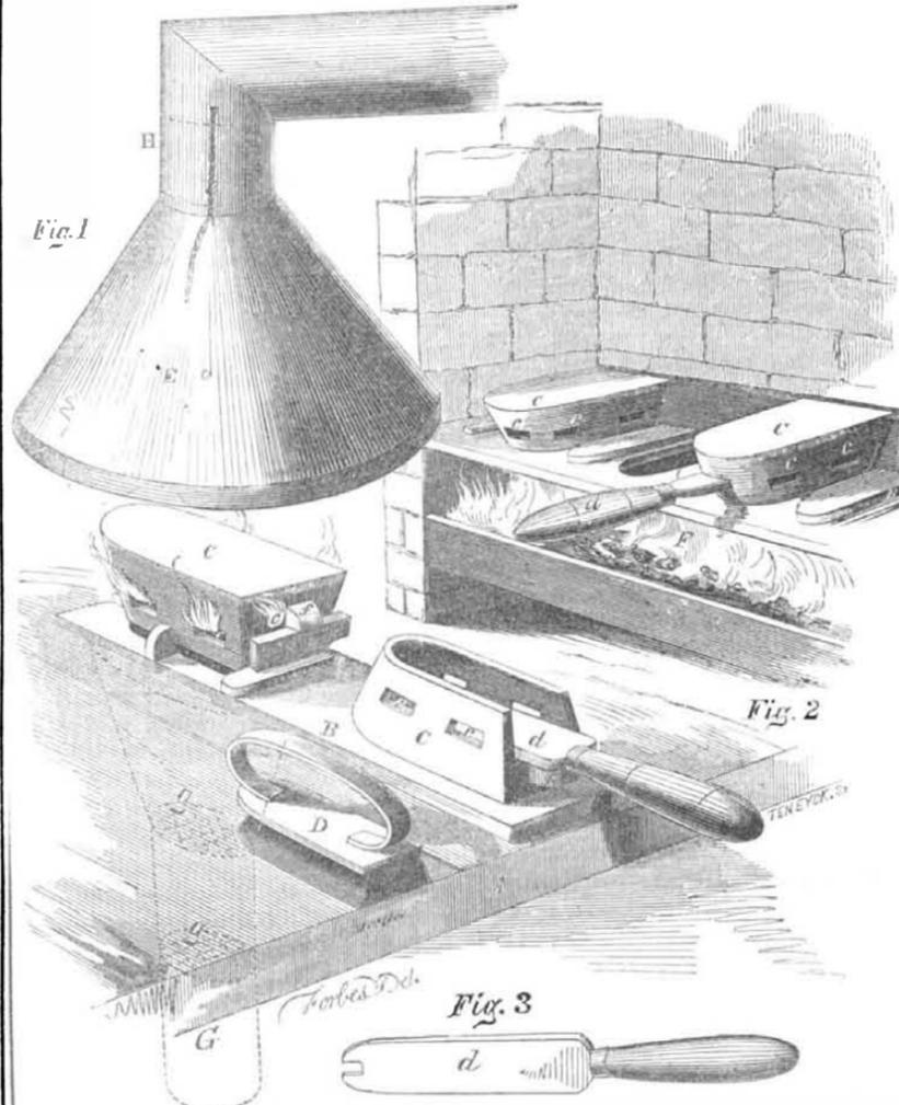
The annexed engravings are views in perspective of new irons, apparatus, and system for heating the irons, invented by L. W. Boynton, of this city, who has taken measures to secure a patent for the same.
