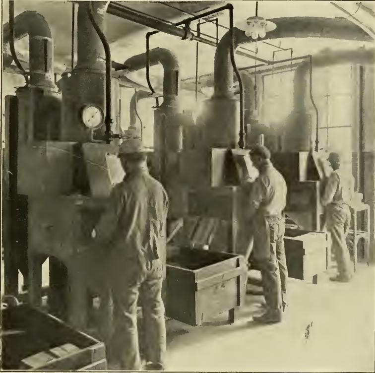
FIG. 16. CABINETS FOR SAND-BLASTING SMALL CASTINGS.
