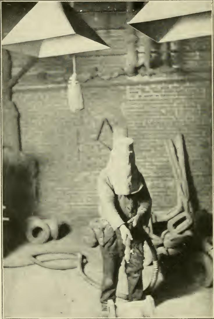
FIG. 15. A SPECIAL CHAMBER FOR SAND-BLASTING.
