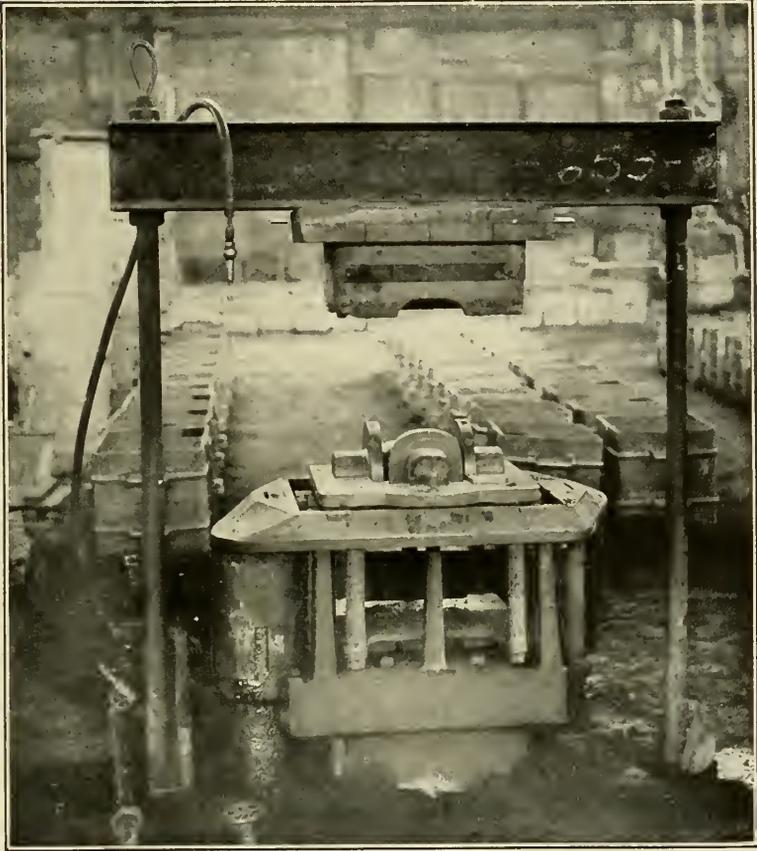
FIG. 14. MOLDING MACHINE OPERATED BY COMPRESSED AIR.
