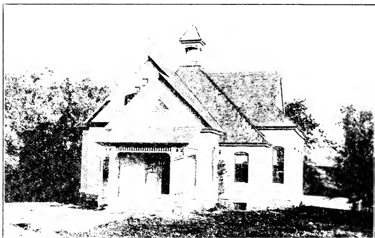
An up to date district school. This School building is being enlarged to accommodate pupils on the Consolidated plan.
