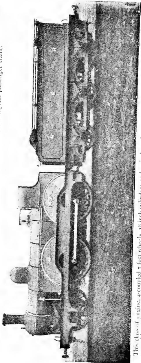
This class of engine, 4-coupled 7 feet wheels, 18 inch cylinders, and 24 inch stroke, was built in 1885, at the time the Company was without the services of a Locomotive Superintendent. The General Manager, Mr. Henry J. Hunt, undertook the direct supervision over the department at that period, and hence these engines are named the "Tennant Express."
