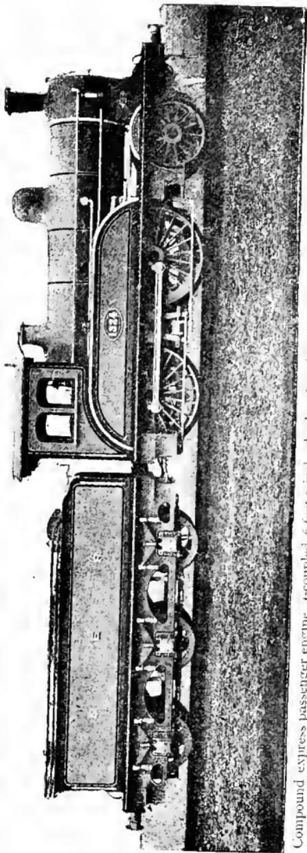
Compound express passenger engine, 4-coupled 6 feet 6 inch wheels, 18 and 26 inch cylinders, and 24 inch stroke, boiler pressure 175 lbs., was designed in 1886 by Mr. T. W. Worsdell for main line express passenger traffic.
