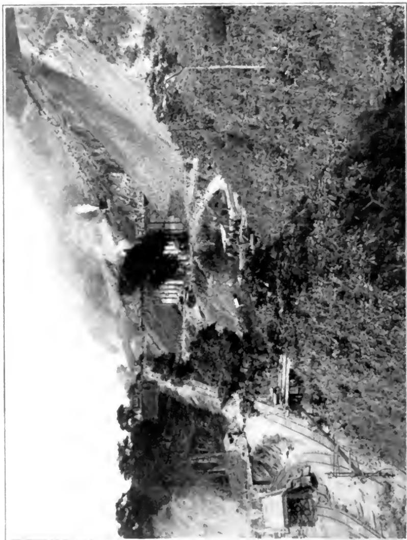
Crushing Plant Installed for United States Government at Ancon Hill, Panama, Consisting of One 36-inch Mammoth and Four No. 6 McCully Crushers.
