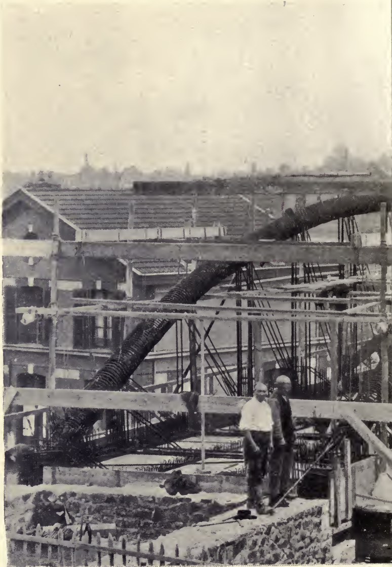
FIG. 80.—RAILWAY BRIDGE OVER THE RIVER SÉE
