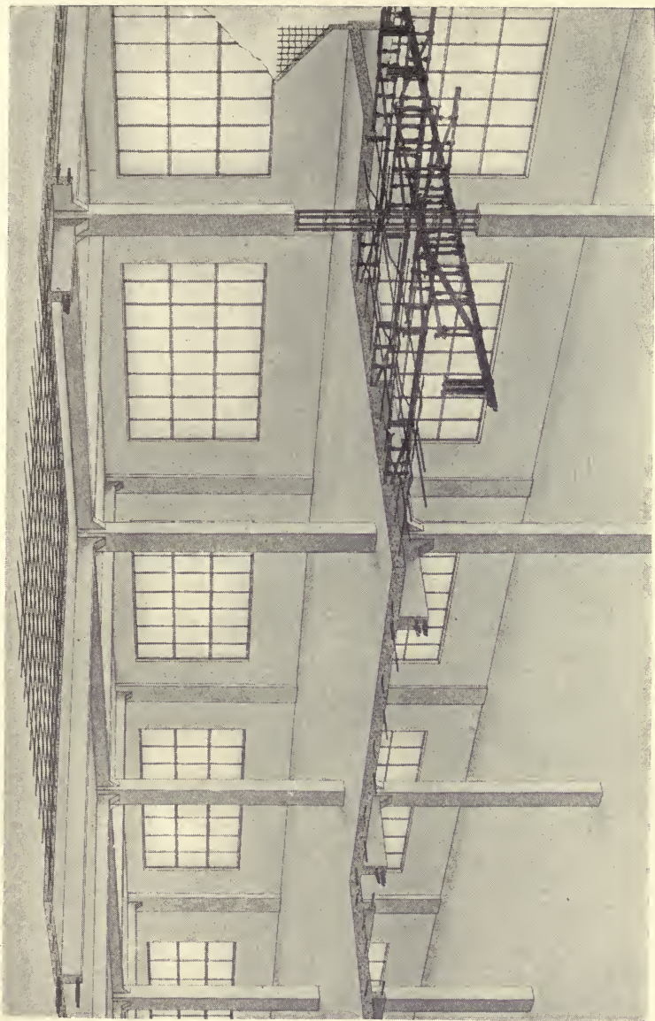
FIG. 191.—VIEW OF FLOOR CONSTRUCTION UNDER THE LESLIE SYSTEM.
