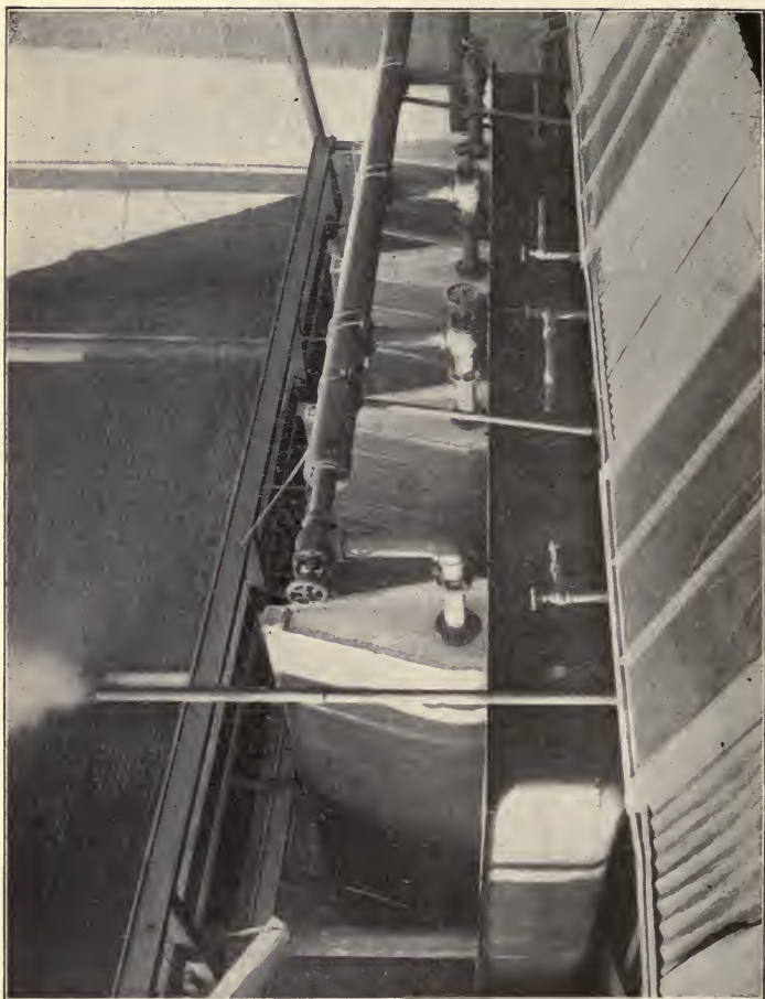
Fig. 60. Triumph Steam Condenser.
