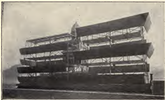
Fig. 46. Cooling Tower Installed at a Large Brewery in Monterey, Mexico.
