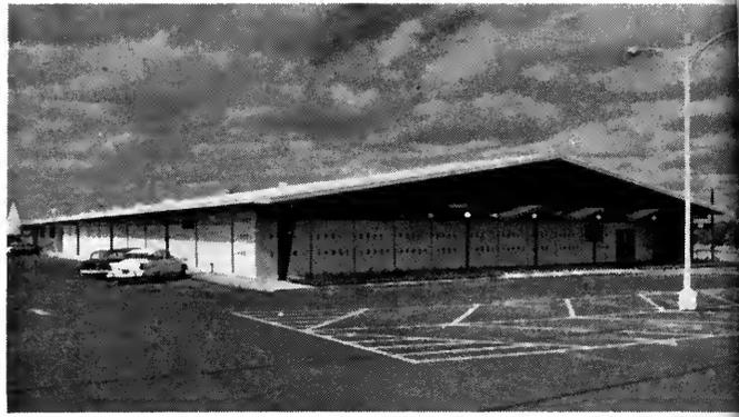
*Westview Playland in Waco, Texas, is housed in a 436-foot-long steel building. Clear span, unobstructed by columns, allows building to accommodate roller skating and play area.*
