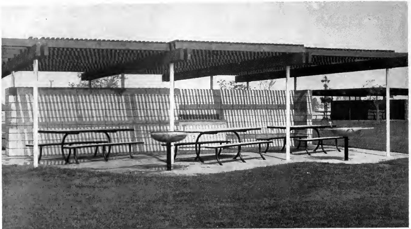
*New picnic shelters are shaded by redwood lathes, feature functional steel-and-concrete table and bench units.*
