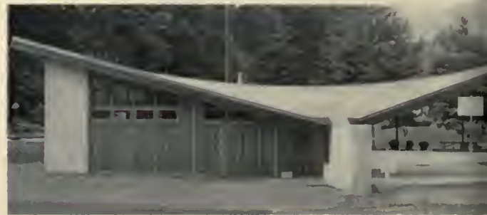
This unusual playground pavilion in Hamilton Park, Fort Wayne, Indiana, has a hyperbolic paraboloid roof, providing a protected outdoor recreation area not hampered by supports. Overall dimension is fifty-six square feet.
