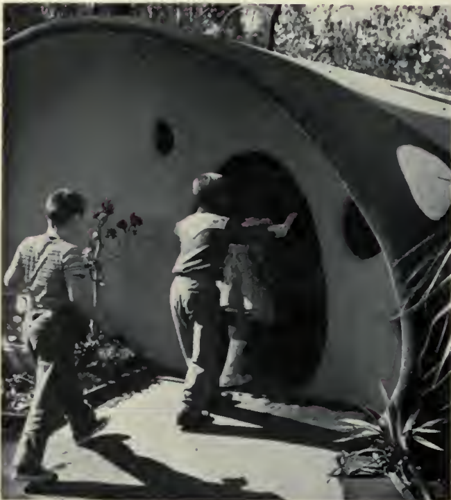
The entrance is just the right height and leads into tunnel where burrowing rodents are displayed. Styrofoam insulation was applied to the expanded metal to protect the animals.
