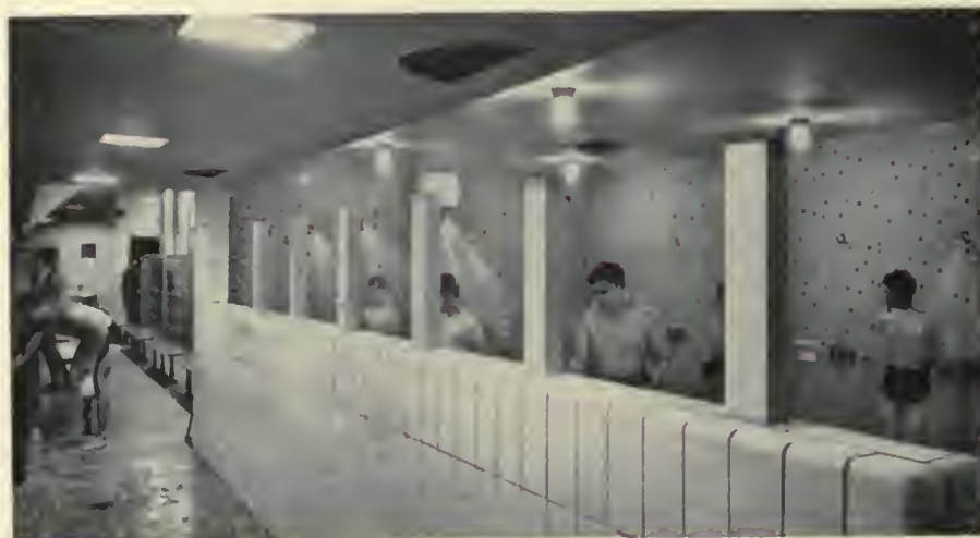
Ceramic-tile walls and floor bring color and maintenance ease to boys' shower room. The low glazed structural-tile partitions allow full shower supervision at all times.
