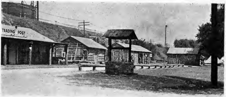
View of one side of the square showing four of the nine buildings. The well in the foreground is equipped with four bubbler drinking fountains
