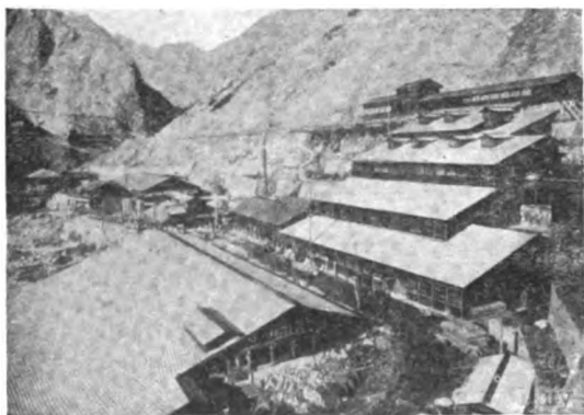
FIG. 81. ORE-DRESSING PLANT, KOTAKI.
