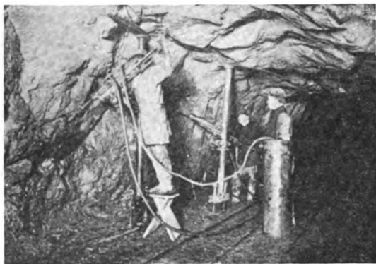
FIG. 80. LEYNER DRILLS AT WORK.
