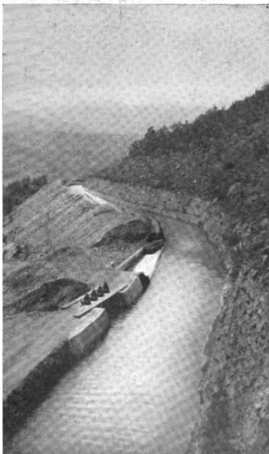
FIG. 51. CANAL GATE SPILLWAY, AND AUTOMATIC SPILLWAY, BRADEN.
