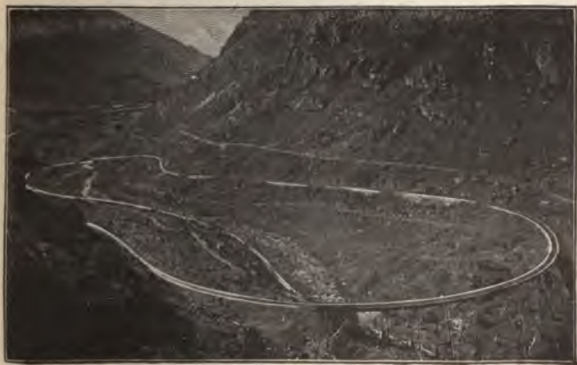
FIG. 102. A railway on an inclined plane in the Rocky Mountains. The altitude is conquered gradually.
