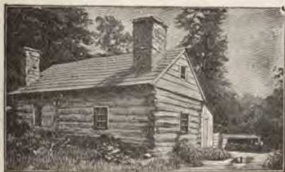
FIG. 377. A log house like those built by the early settlers of America except that those had no glass windows. Chimneys were at first built of stones or clay, afterwards of brick. The first bricks in America were brought in ships from England. But as the colonists perfectly understood how to make and burn bricks it was not very long before they made all that were needed.
