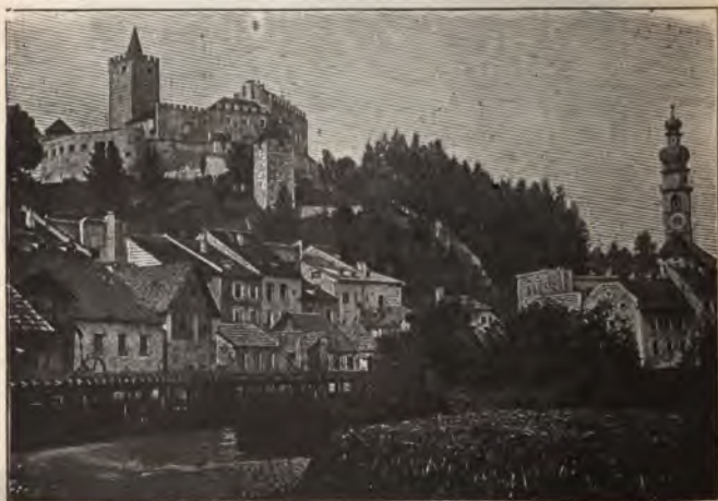
FIG. 384. A castle in Austria, built in the middle ages (before the fifteenth century). Notice its thick walls made for defence.
