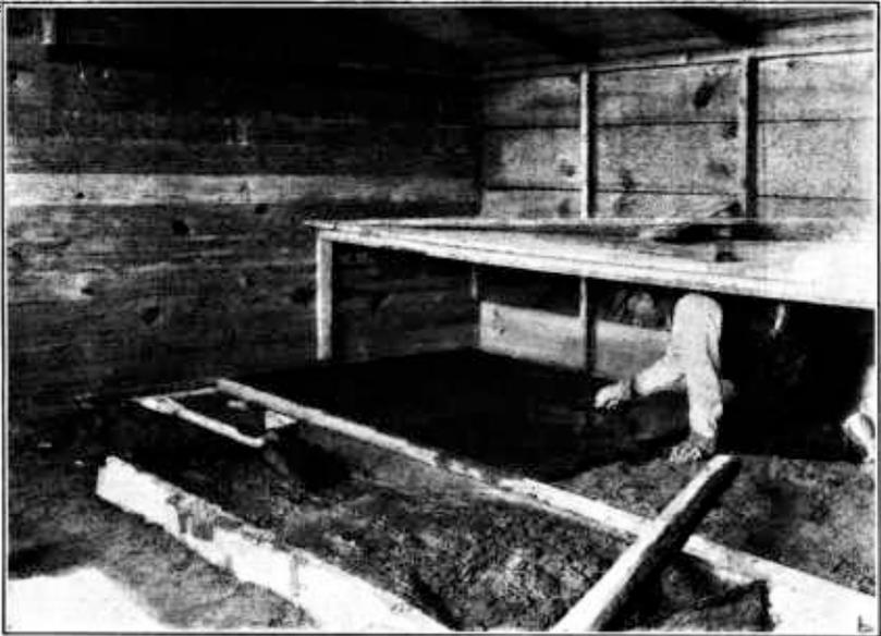
FIGURE 13.—Rat proofing a poultry house by laying a concrete floor
