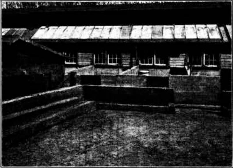
FIGURE 11.—Rat-proof pigpens and feeding troughs are easy to keep clean and sanitary, and rats have little opportunity to steal the feed B4390M
