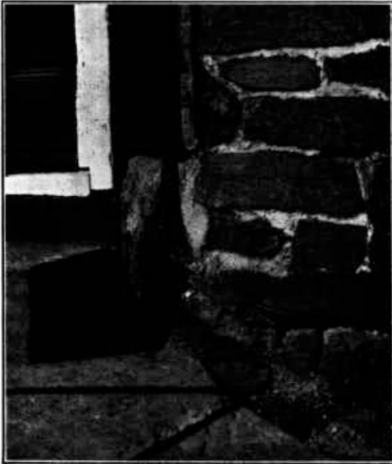
FIGURE 19.—Defects in foundations, such as the opening to the right of the step, are often the cause of rat infestation in old buildings
