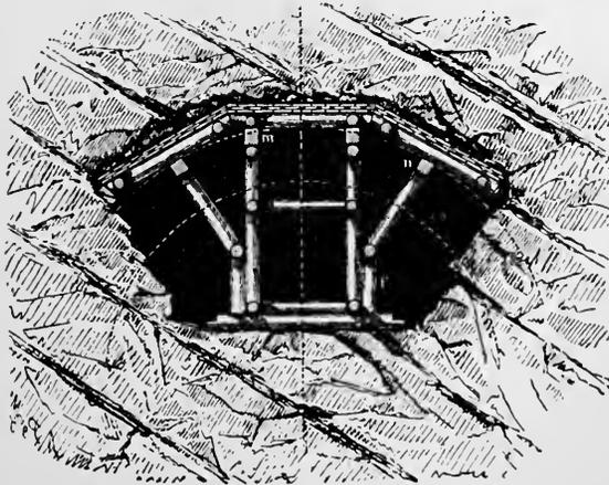
TUNNEL-TIMBERING—AUSTRIAN SYSTEM (c).
