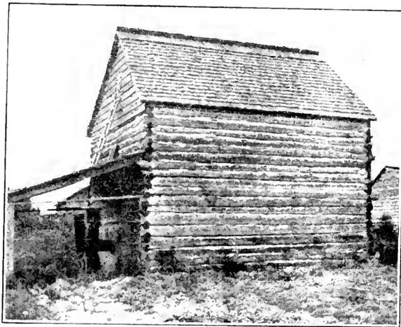
FIG. 8.—A typical log barn used in curing yellow tobacco, showing the ventilator in the gable and the outside portions of the heating system.
