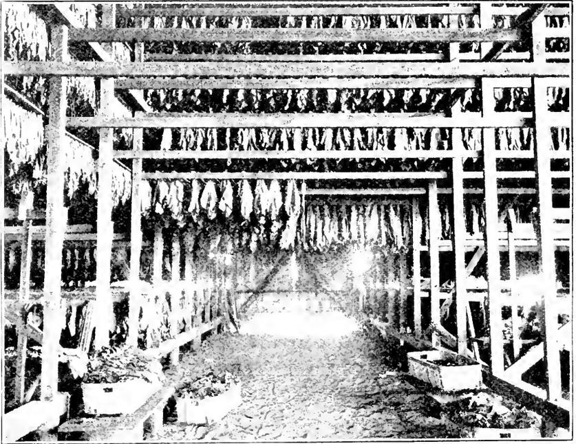
FIG. 6.—The interior of a cigar-tobacco barn, showing the arrangement of tier poles and the method of hanging picked leaves.
