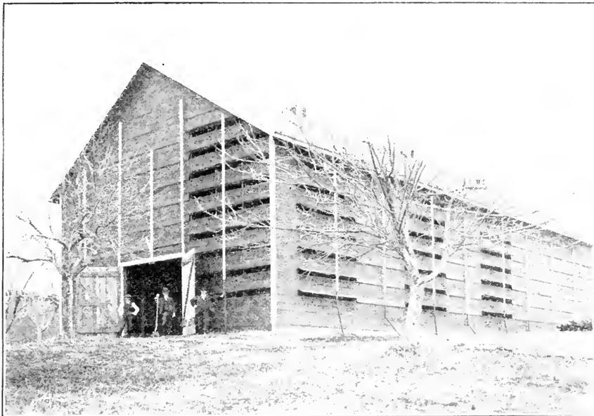
FIG. 1.—Type of barn used in northern cigar-tobacco districts, showing the arrangement of horizontal ventilators.
