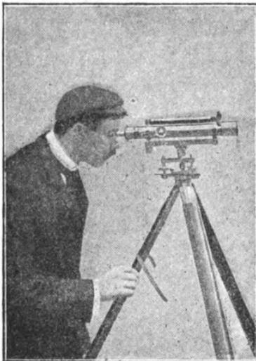
FIG. 129.—How NOT to use a level.
