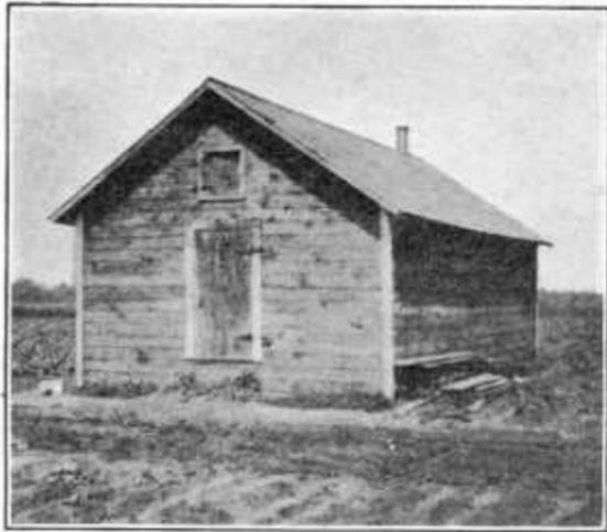
FIGURE 15.—An insulated frame potato-storage house used for storing second-crop potatoes. Morrill, Tex.
