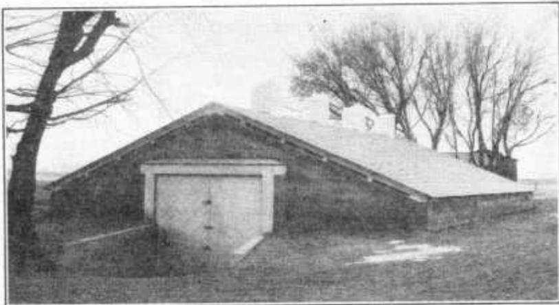
FIGURE 10.—Dugout potato-storage cellar with straw and soil roof and superimposed water-tight roof. Greeley, Colo.
