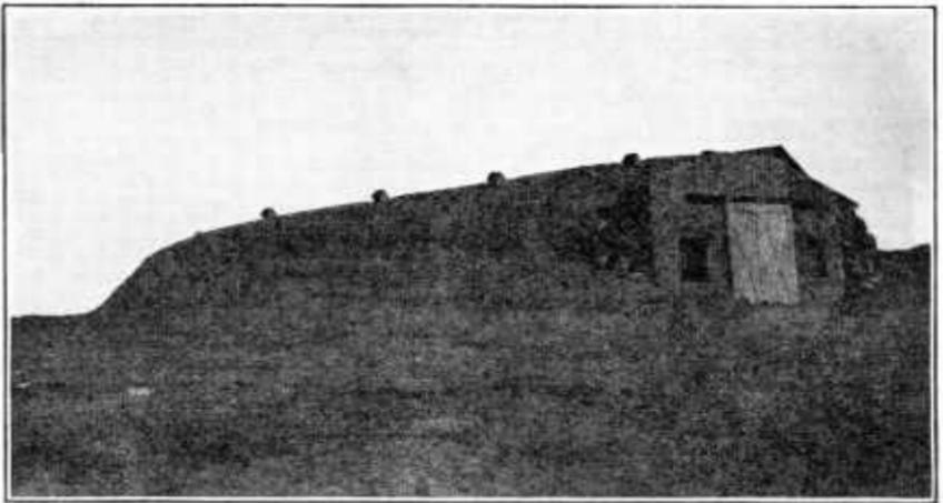
FIGURE 18.—Former potato-storage cellar of the U. S. Department of Agriculture at Jerome, Idaho, showing end entrance and arrangement of ventilators
