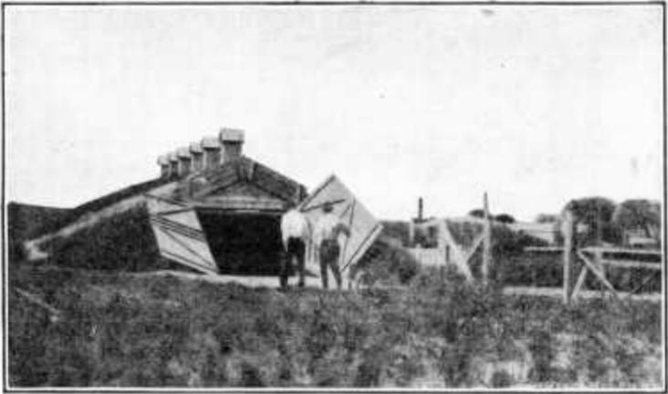
FIGURE 11.—A potato-storage cellar, showing a bulkhead driveway entrance in which the grade into the cellar is provided inside the entry to the bulkhead. Jerome, Idaho
