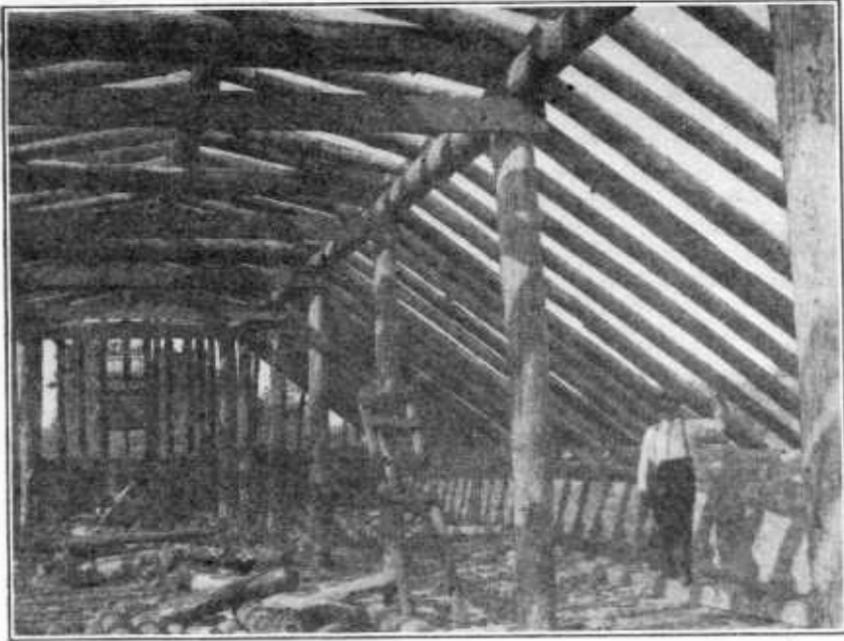
FIGURE 9.—Interior view of a potato-storage cellar with side and end walls of stone, showing the type of roof construction used. Greeley, Colo.
