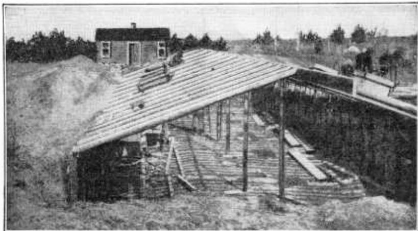
FIGURE 6.—A potato-storage house in course of construction, showing posts recessed in walls of earth and the method of placing ventilators in the roof, Jerome, Idaho
