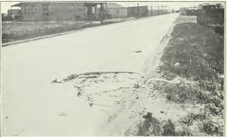
FIG. 2.—FAILURE OF A THIN CONCRETE PAVEMENT UNDER HEAVY TRAFFIC.
