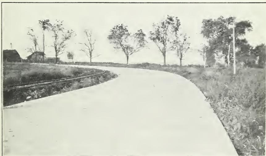
FIG. 2.—SUPER ELEVATED CURVE BEFORE THE CONSTRUCTION OF THE
