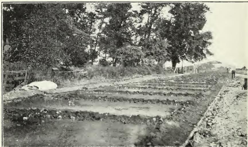
FIG. 2.—THE PONDING METHOD OF CURING.
