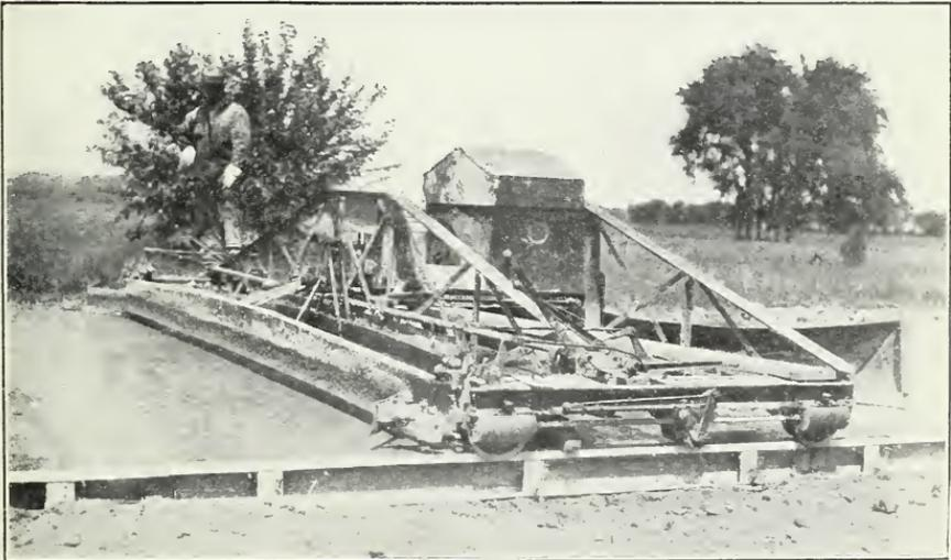
FIG. 2.—MECHANICAL FINISHING MACHINE FOR CONCRETE PAVEMENTS.
