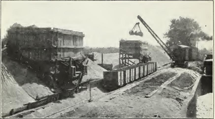
FIG. 1.—LOADING BATCH BOXES FROM OPEN BINS.
