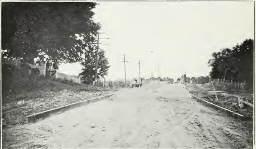
FIG. 2.—FINE AND COARSE AGGREGATE PILED ON SUBGRADE READY FOR USE.
