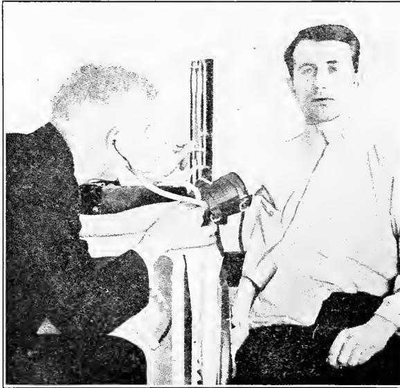
Fig. 130.—Observation by the auscultatory method and a mercury instrument. One hand regulates the stopcock which releases air gradually. (From Warfield.)
