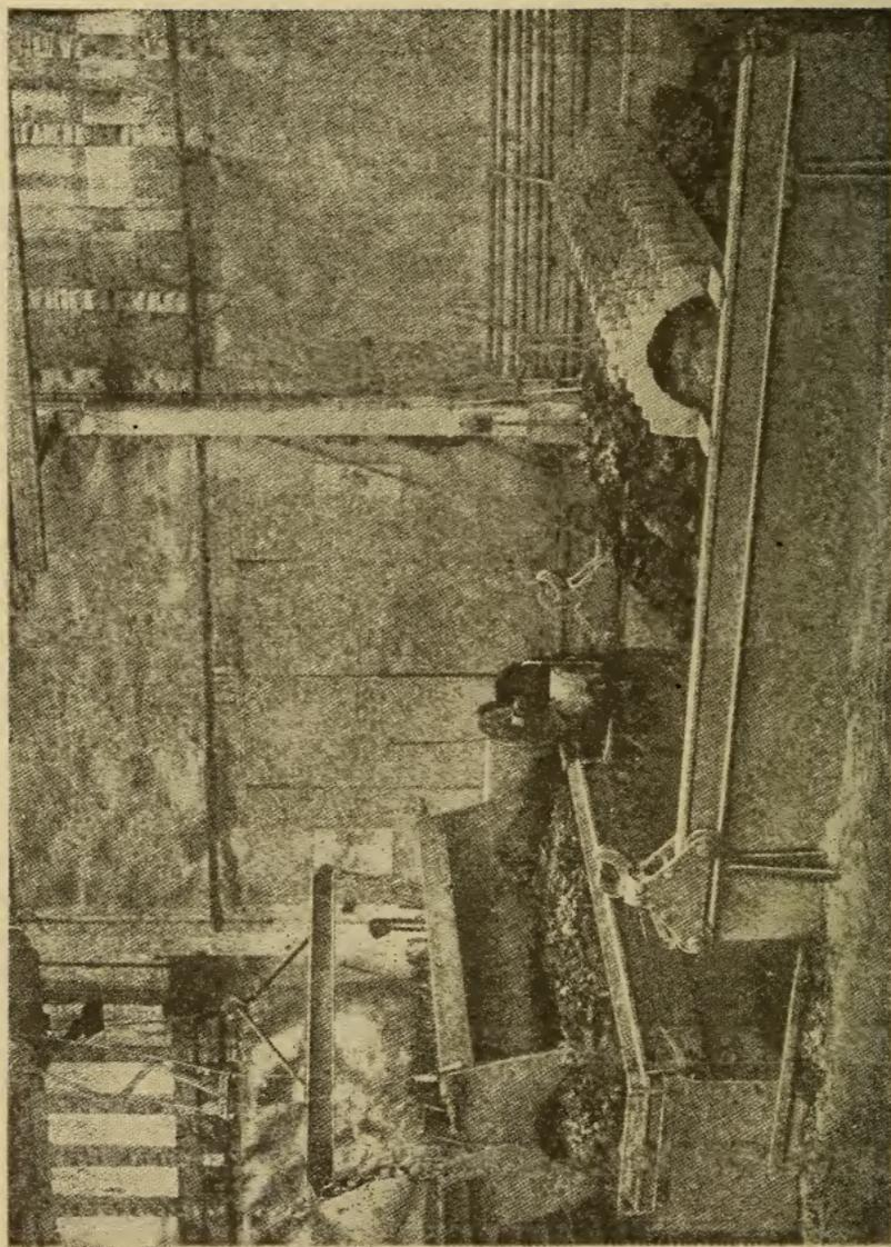
**MOLDAR SAND SHOVEL DEPOSITING SAND IN FLASK**
