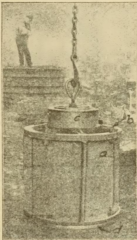
Fig. 376. Pattern Being Drawn through Stripping Ring
