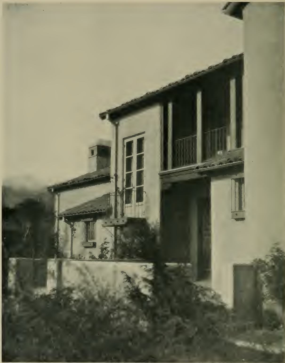
MAIN ENTRANCE DETAIL
