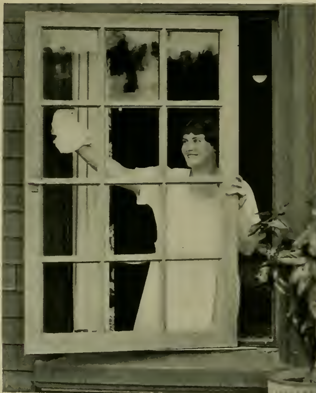
The windows fully reverse. Both surfaces are cleaned from the inside of the room.
