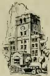
Bell Tower Kohler Administration Building
