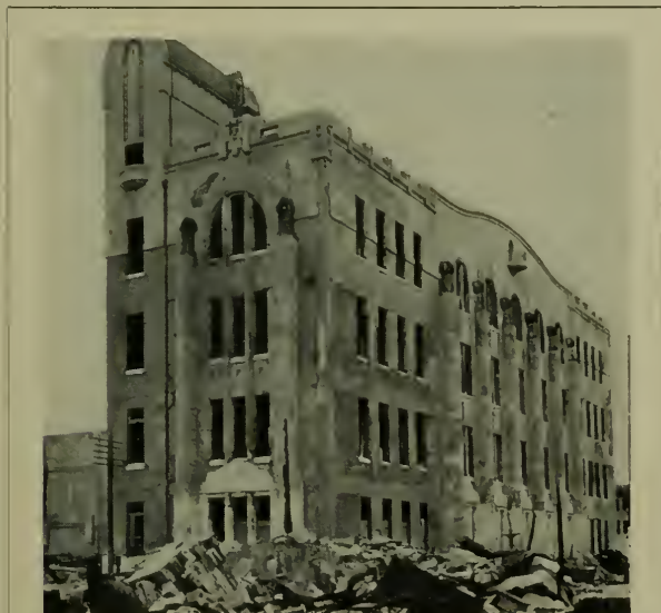
YOKOHAMA TELEPHONE BUILDING. TALLEST BUILDING IN YOKOHAMA. DAMAGED BY SKELETON CONSTRUCTION BUILDING LACKED STIFFNESS IN NARROW DIRECTION
