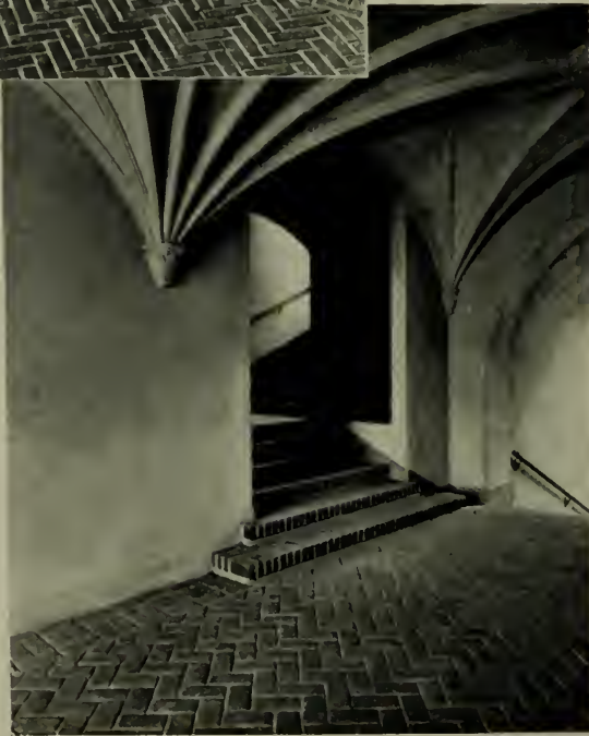
TOWER STAIRWAY STUDENTS UNION BUILDING UNIVERSITY OF CALIFORNIA THE STRUCTURE ITSELF IS BUILT OF DICKY MASTER TILE — ARCHITECT: JOHN GALEN HOWARD — MASONRY CONTRACTOR: N. B. MCGOWAN
