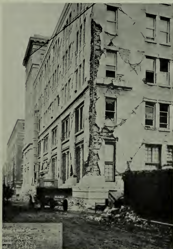
TOP: STEEL FRAME BUILDING SHOWING COMPARATIVELY UNIMPORTANT DAMAGE. LOWER LEFT: RUSSO ASIATIC BANK, TOKIO, REINFORCED CONCRETE STRUCTURE. LOWER RIGHT: JAPAN OIL BUILDING, TOKIO, STEEL FRAME STRUCTURE, FACED WITH TERRA COTTA, BACKED WITH COMMON BRICK
