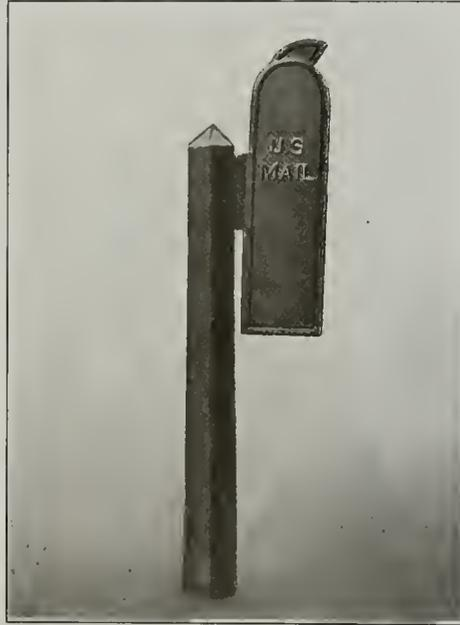
of reinforced concrete and will prove permanent; they are of hexagon shape, 8 inches in diameter at the bottom, tapering to 6 inches at the top;  $4\frac{3}{8}$ -inch iron rods, tied with strong wire, are used for the reinforcement.
