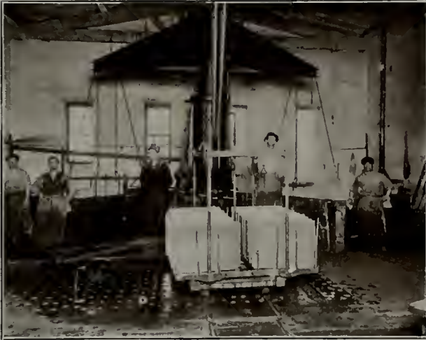
Pickling department, N. & G. Taylor's, Cumberland, Md., works. Here the black sheets are cleaned with a weak solution of acid and thoroughly washed in clean water before being transferred to the various tinning stacks. These black plates are a special quality made at the Taylor works from the pig iron through to the finished sheet.
