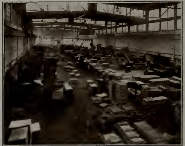
General view of new tinning department, showing the excellent lighting facilities. All handling of material done by overhead traveling crane. The tinning stacks are located in the recesses along either side of the building.
