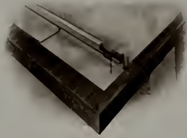
FIG. J.—STANDING-SEAM TIN ROOFING Fourth operation. Standing seam completed, showing cleat in position. Thickness of seam magnified, to show the folds of the metal.
