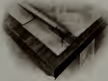
FIG. H.—STANDING-SEAM TIN ROOFING Third operation. Entire seam turned partly over.
