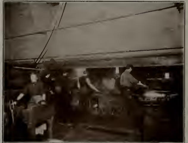
The full "seven open pot, palm oil, hand dipping stack," an exclusive process employed only by the N. & G. Taylor Co. Used only in making the Target and Arrow brand of roofing tin. This is the old time process formerly employed in the company's works in Wales. All work done by hand, four skilled workmen being required. By this process the coating is slowly and thoroughly applied in successive layers on the sheet, resulting in an exceptionally durable roofing plate.
